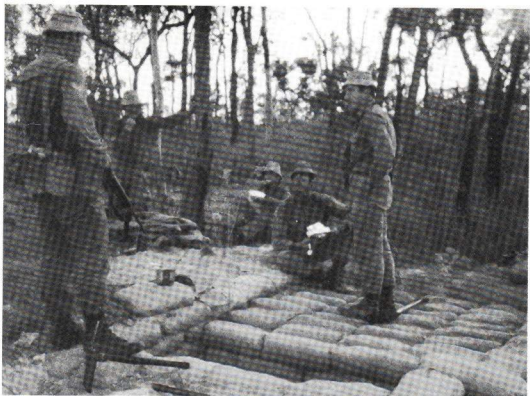
The 2IC on top of the bunker.
